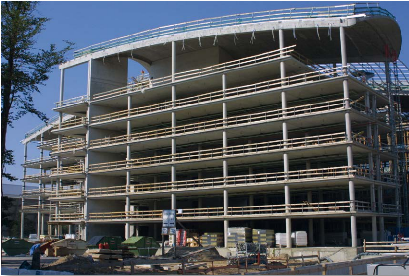
Figure 4: Column structure of the Lufthansa Aviation Centre in Frankfurt
