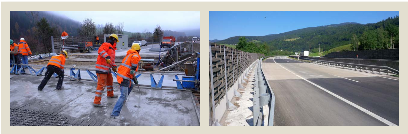
Figure 21: Work on bridge strengthening with UHPC at the Steinbach bridge, Austria
