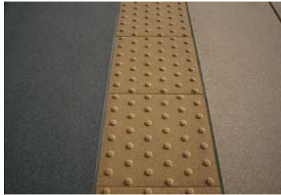
Fig. 2 Result: the completed platform unit.
